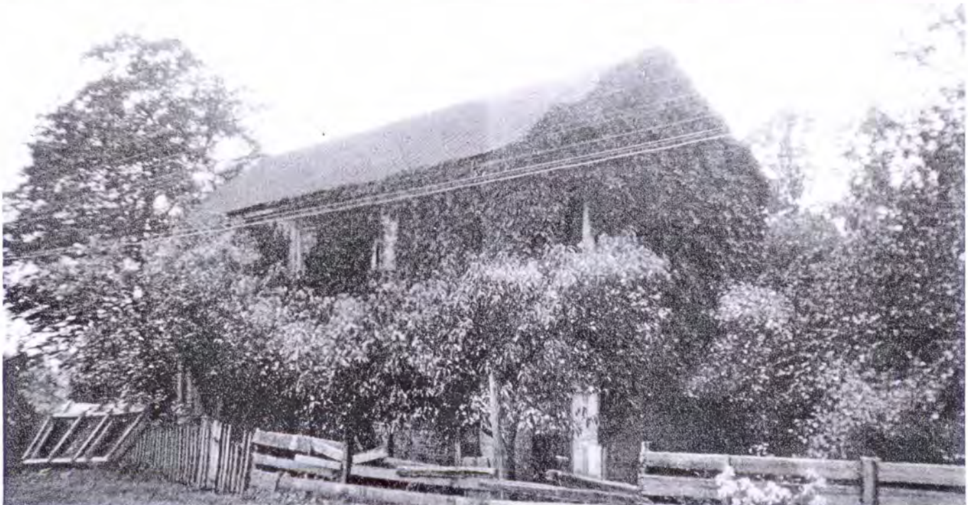
This portion of the McMurdy School is still standing in Washington
